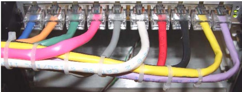
**FIGURE 1-19 FE10 RJ45 Connector Dressing**
