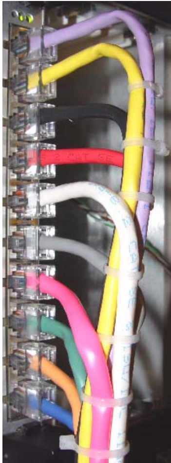
FIGURE 1-23 FE10 RJ45 Connector Dressing
